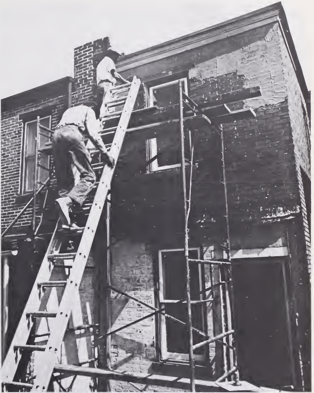
CHIP REHABILITATION IN PROGRESS
